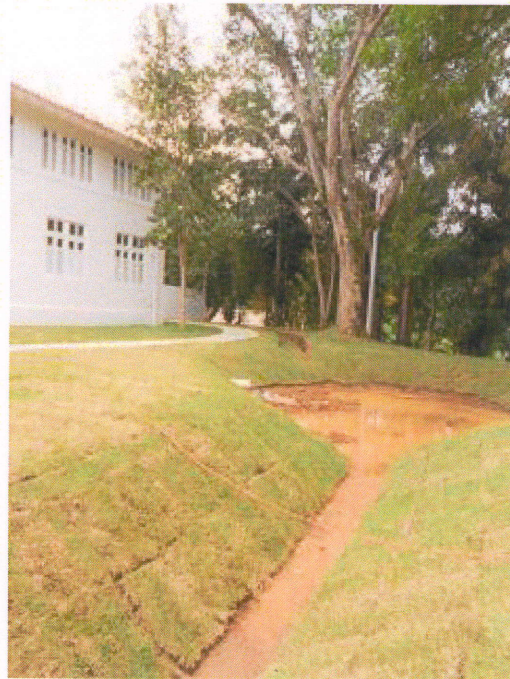
This detention pond on the grounds of the International Institute for Tropical Forestry in Puerto Rico will help reduce flooding of nearby neighborhoods. Photo by Melanie Lenart
